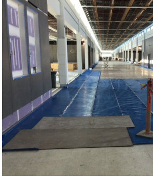
Airport Terminal; New Terrazzo Floor Protection
