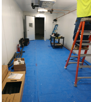
Interior Electrical Renovation; Floor Protection
