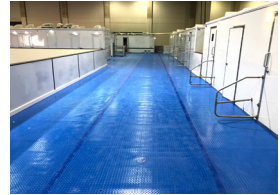
COVID Field Hospital; Temporary Flooring
