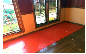
Home Renovation; Hardwood Floor Protection
