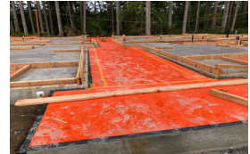
Outdoor Application; Concrete Protection
