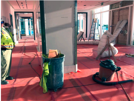
Commercial New Construction; Floor/Column Protection
