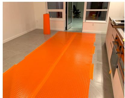
Commercial Renovation; Corridor Floor Protection
