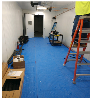
Interior Electrical Renovation; Floor Protection
