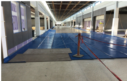
Airport Terminal; New Terrazzo Floor Protection
