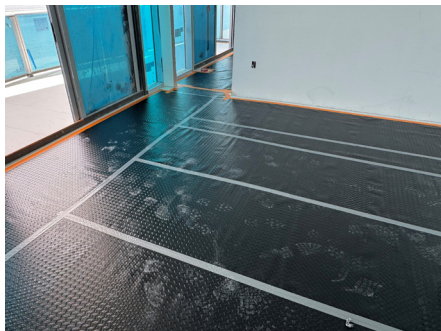
Commercial New Construction; Floor Protection
