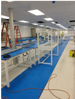
Industrial Lab; Floor/Counter Protection
